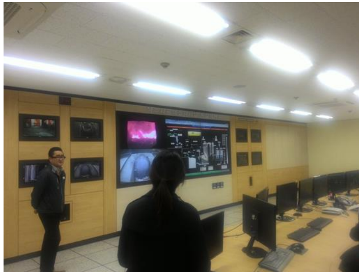
View inside the monitoring room.
